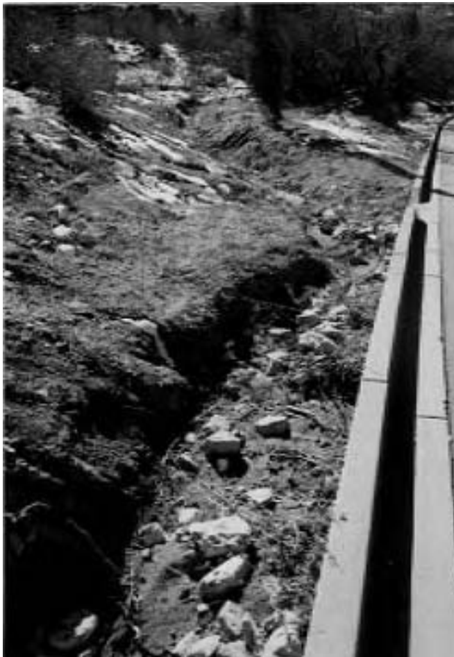
Examples of the erosion occurring along the edges of the roadways in the Park.
