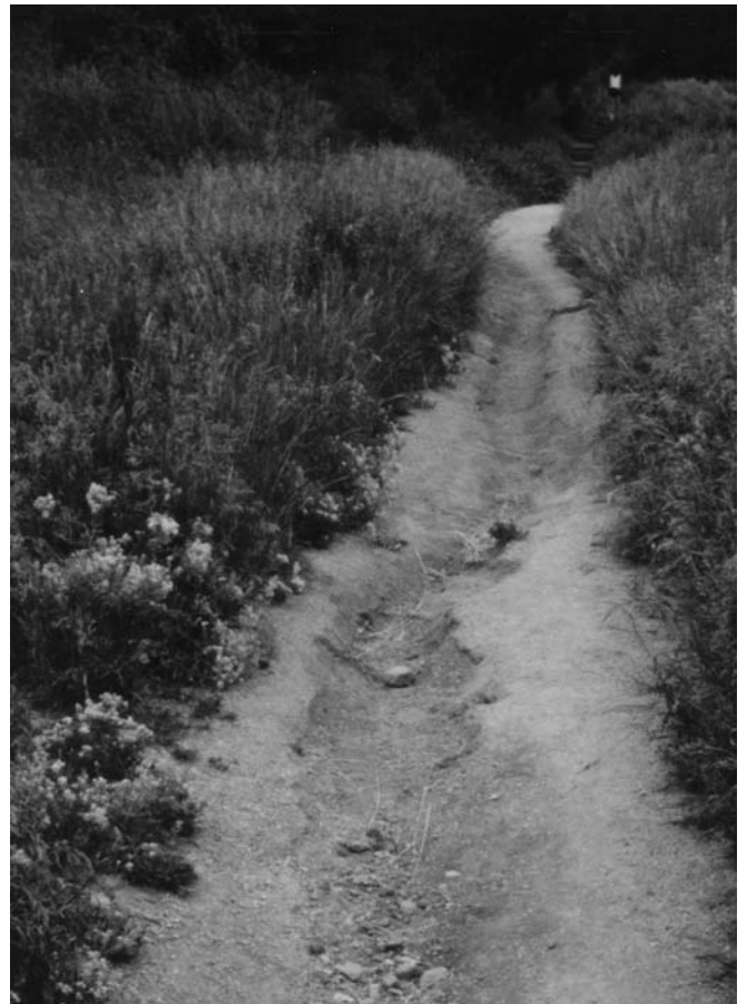
Example of Class 3 Trails: 7-12 inches of soil loss.
