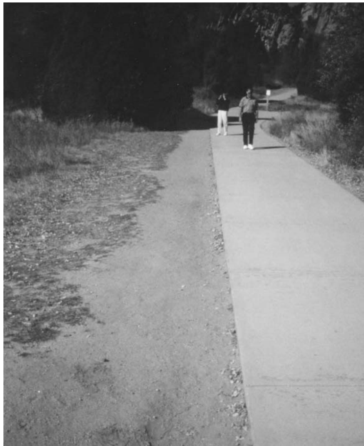
Erosion (Class 3) along the edge of paved (concrete) walkway in central Garden zone.
