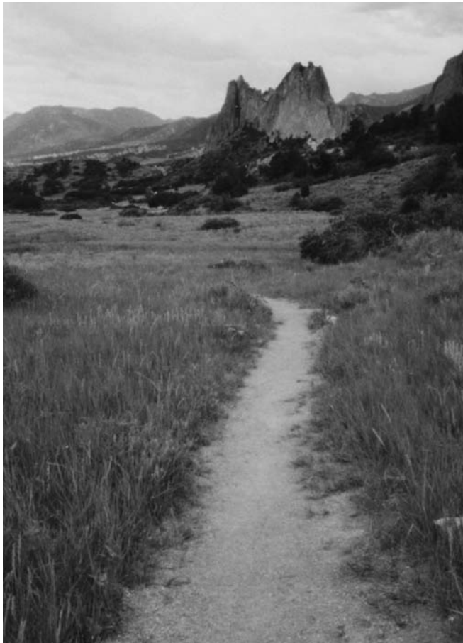
Example of Class 2 Trails: 1-6 inches of soil loss.
