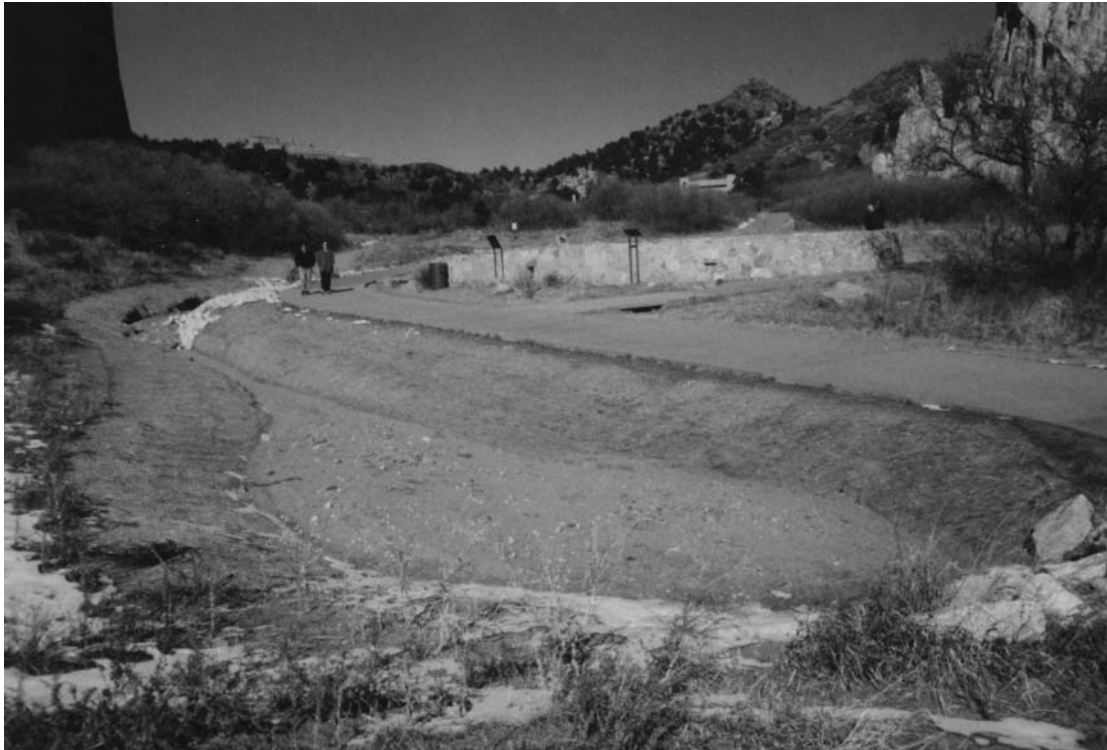
This photo shows the drainage gully on the east side of North Gateway (Kissing Camels Rock). A sewer line for the toilets near the parking lot was installed, but the site was not fully restored. A gully of this size never existed at this location.
