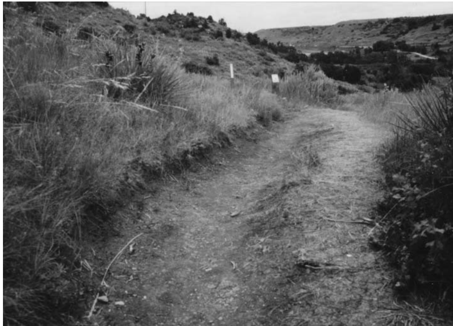
Example of Class 4 Trails: More than 12 inches of soil loss.
